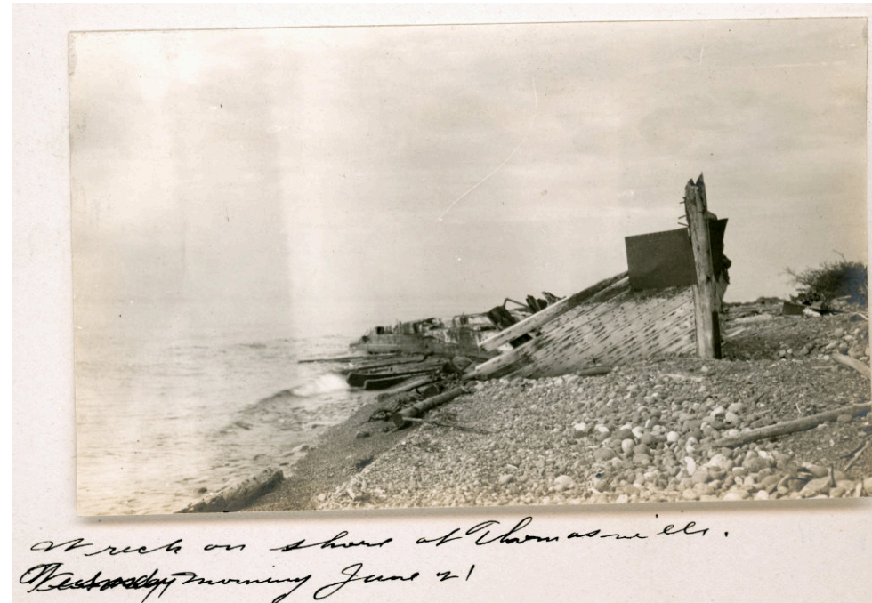
Wreck on shore of Thomasville. Wednesday morning June 21
