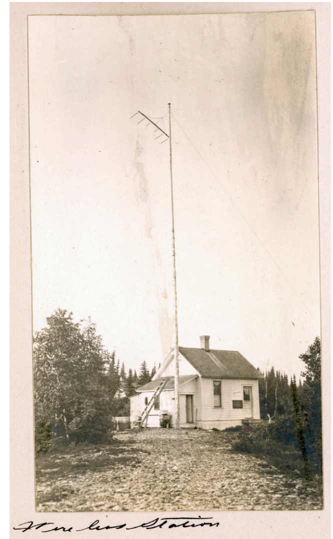
Wireless Station (Grand Marais)
