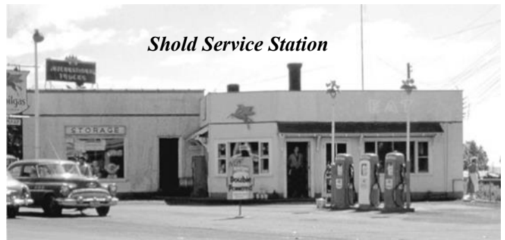
The Kaffe Stuga was located in right side of the building. The "lube" wing is on the left. c1950
